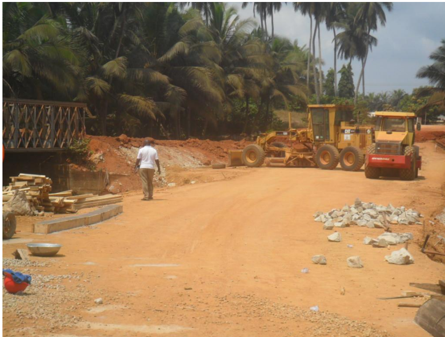
Figure 13: A new bridge under construction over Ellonu lagoon
